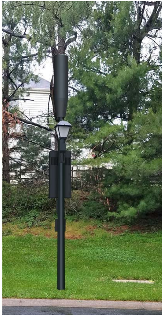
14' to 16' Colonial Streetlight Replaced with 19' to 20' side mounted or ground cabinet
